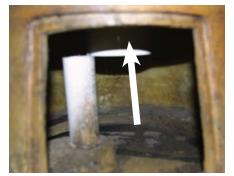
Inside of pedestal with PVC screw attached.
